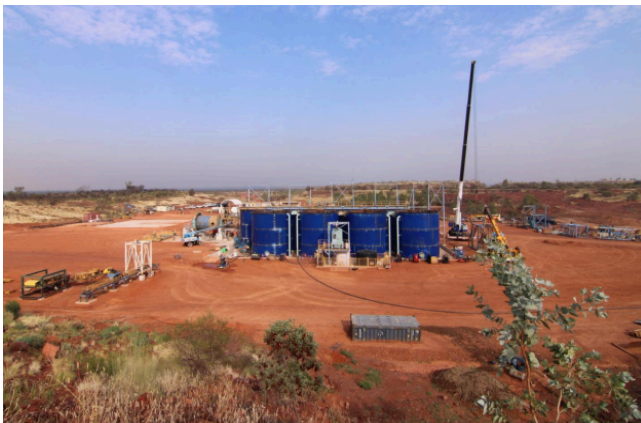
Figure 4: Nobles Plant Under Construction
