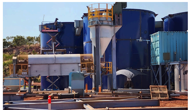
Figure 5: Nobles Plant Under Construction
